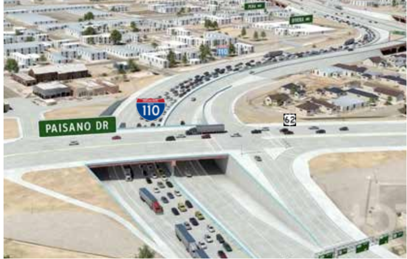
Complete reconstruction of the I-110/US 62 (Paisano Drive) interchange including removal of ramps from Paisano Drive to the Bridge of the Americas.
